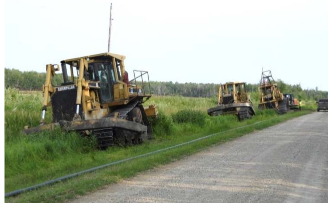
Equipment trenching in water pipe.
